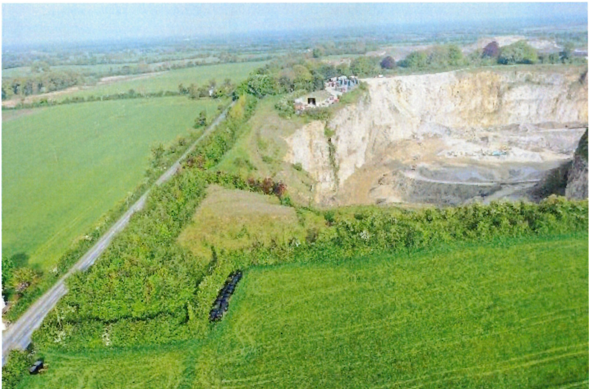
The Road [R156] to the left of the quarry. Note the proximity of the quarry to the road. They were required not to quarry within 60m of the road. This was ignored.
