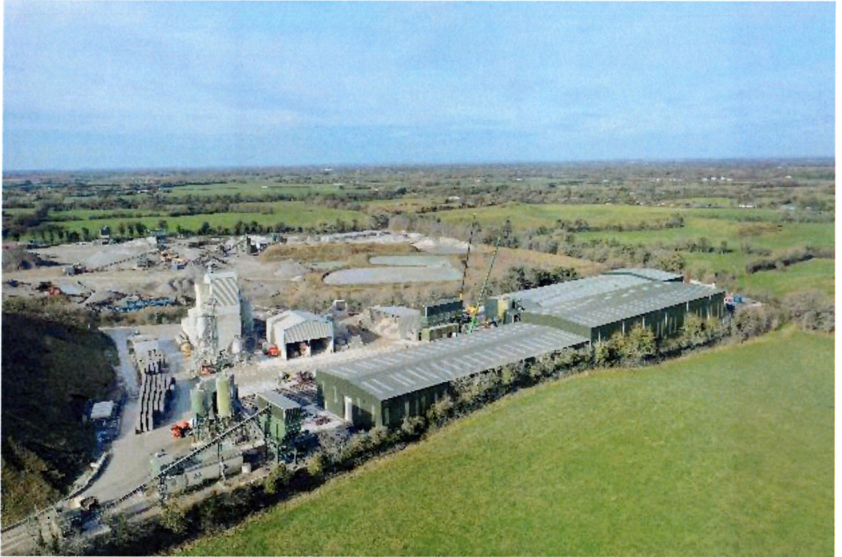
The majority of the structures in this frame were constructed without planning consent.
